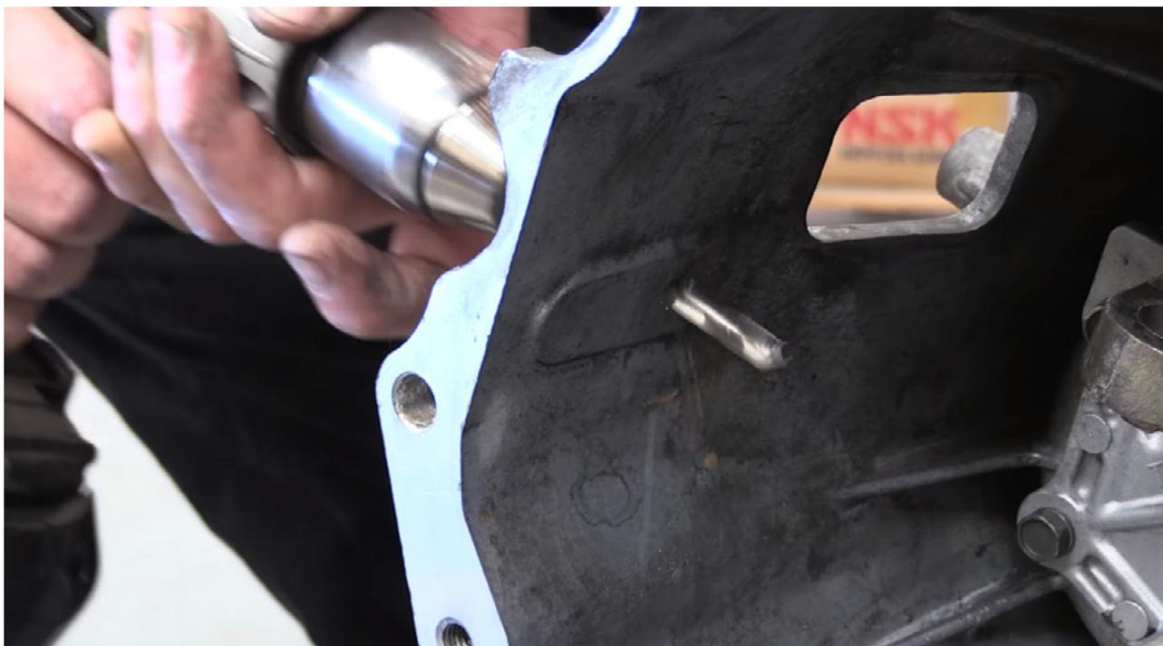
3. Using an 8.5mm drill bit, carefully drill the first hole for the slave. Ensure that the hole is square to the casting surface.
