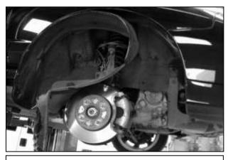
c. Partially remove the splashguard and tuck it out of the way.
