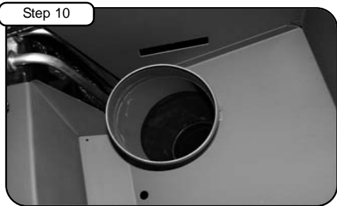
Position housing onto reducer coupler.
