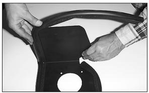
13. Install the trim seal onto the heat shield. NOTE: some cutting and trimming will be necessary to achieve best fit.
